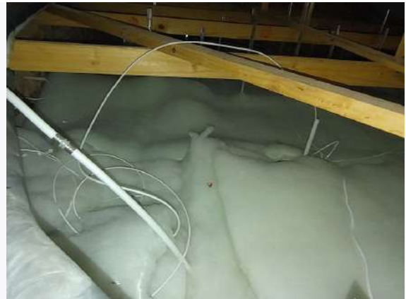
Ref # 5.3 - Roof insulation
