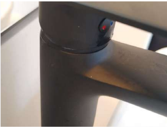
Ref # 18.5 - Mixer has scuff marks
