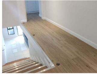
Ref #14 - Image of area inspected
