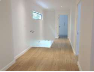
Ref #14 - Image of area inspected
