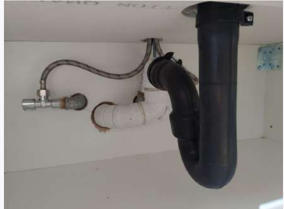
Ref # 20.3 - Image of area inspected
