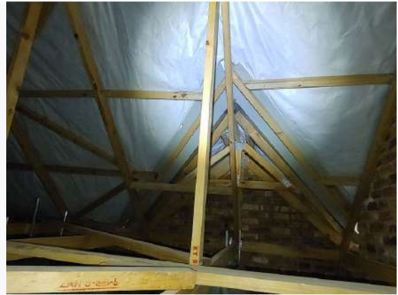
Ref # 5.2 - Roof underlay sheeting
