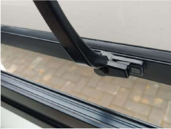
Ref # 15.2 - Window opener loose and requires adjustment
