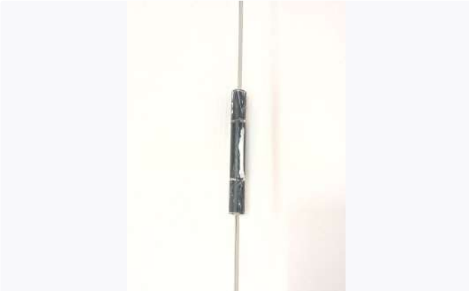
Ref # 18.3 - Untidy finishing
