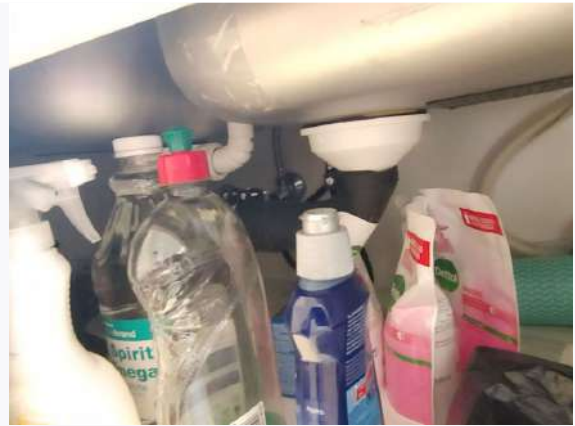
Ref # 16.2 - Image of area inspected
