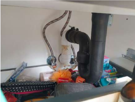
Ref # 18.5 - Image of area inspected
