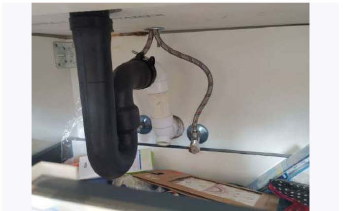
Ref # 18.5 - Image of area inspected
