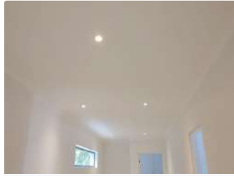
Ref #14 - Image of area inspected
