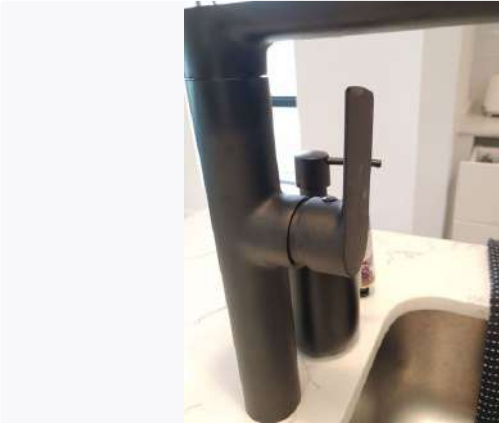
Ref # 16.3 - Mixer has scuff marks and chips
