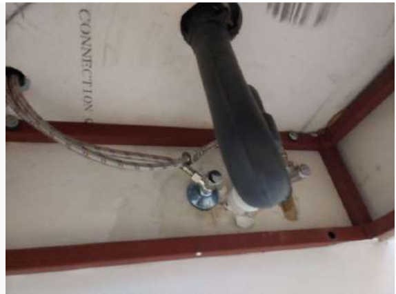
Ref # 21.4 - Image of area inspected
