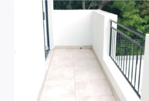
Ref # 10.2 - Verify floor slope directional flow for drainage
