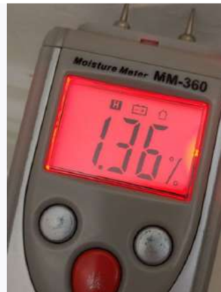
Ref # 21.1 - Active rising / lateral damp measured
