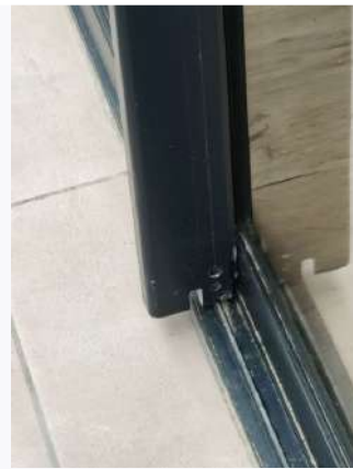
Ref # 12.2 - Sliding door not sliding smoothly
