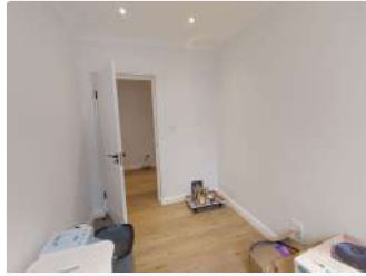
Ref #13 - Image of area inspected
