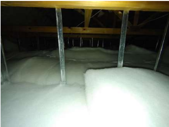
Ref # 5.3 - Roof insulation
