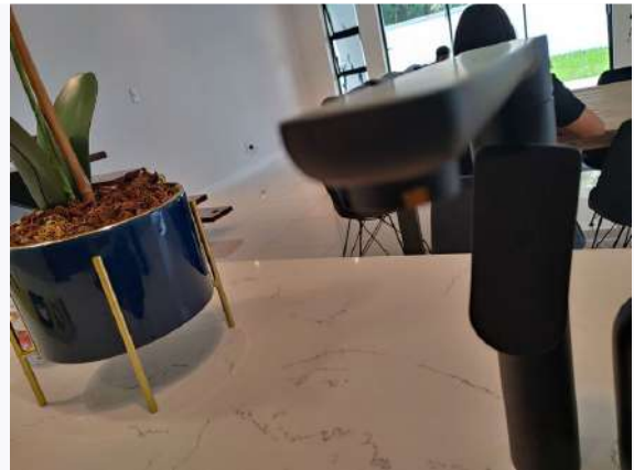
Ref # 16.3 - Mixer has scuff marks and chips
