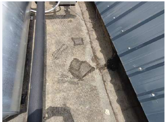
Ref # 4.2 - Remedial work done to waterproofing
