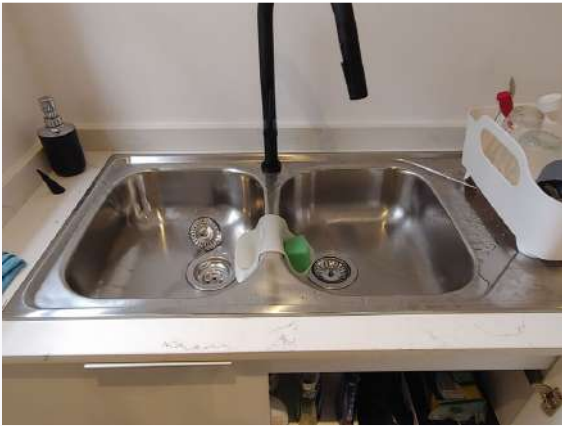
Ref # 16.2 - Image of area inspected
