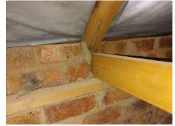
Ref #5 - Truss anchor
