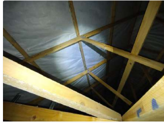
Ref #5 - Roof Cavity
