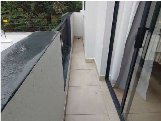
Ref # 12.1 - Verify if the balcony had been waterproofed
