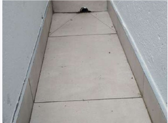
Ref # 12.1 - Verify floor slope directional flow for drainage
