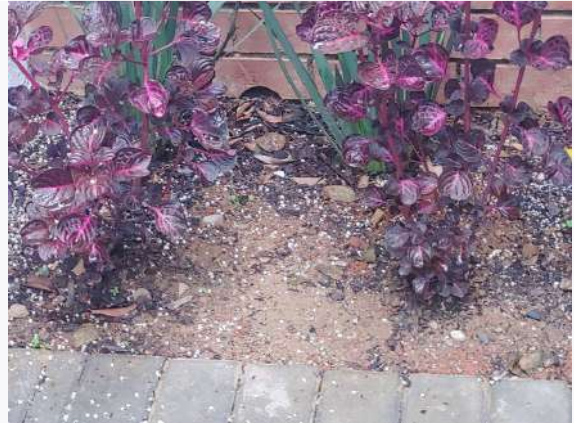
Ref # 23.3 - Weep holes for water run-off drainage is blocked
