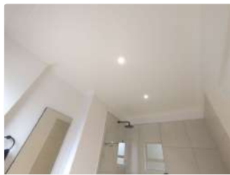
Ref #20 - Image of area inspected
