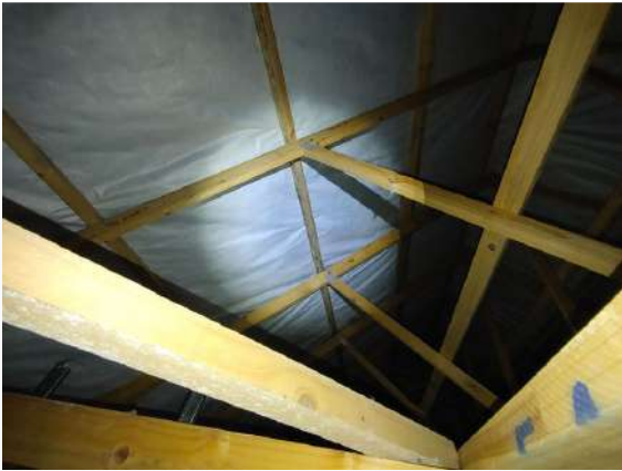
Ref # 5.2 - Roof underlay sheeting
