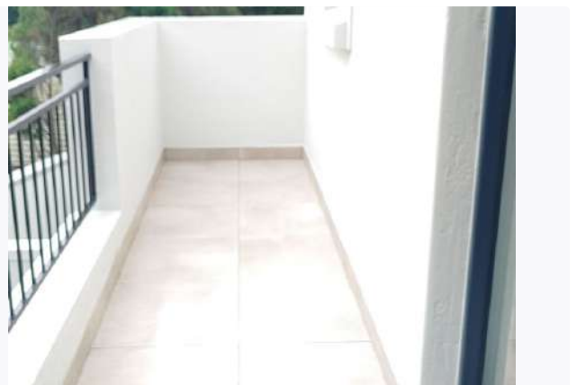
Ref # 10.2 - Verify if the balcony had been waterproofed
