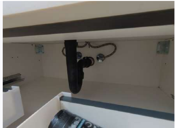
Ref # 19.2 - Image of area inspected
