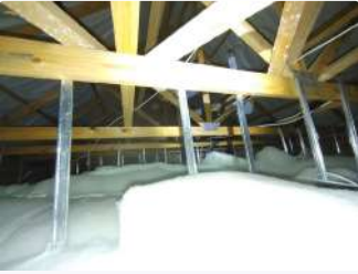
Ref #5 - Roof trusses
