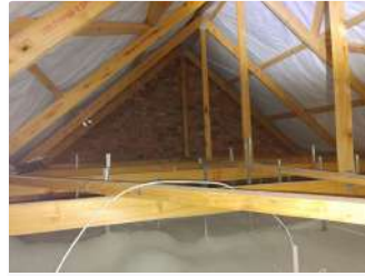
Ref #5 - Roof trusses
